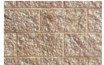
CMU W/GRAFFITI COATING
